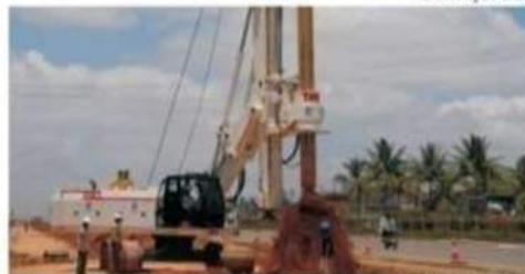
Hydraulic Piling Rig
