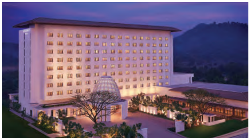
A 150-keys five Star Hotel project for a hospitality major – designed and built by Shapoorji Pallonji E&C
