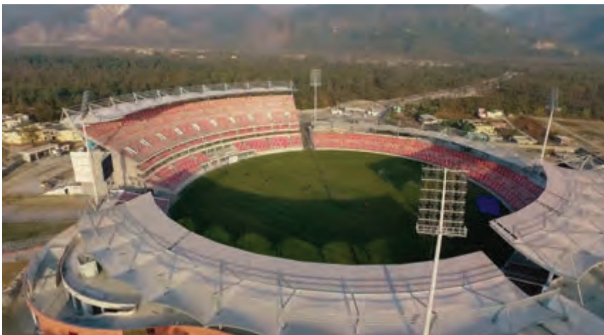
Rajiv Gandhi International Cricket Stadium & Sports Complex at Dehradun – A 25,000 seats capacity stadium, designed and built using precast technology
