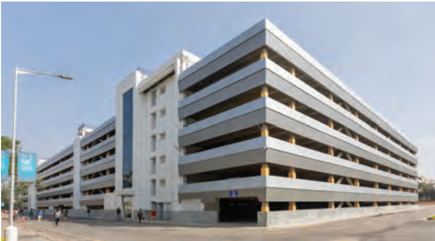
A Multi-Level Car Park of 2,200 cars capacity, designed and built using pre-engineered structural steel
