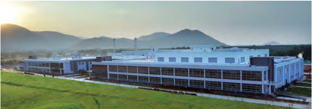
A manufacturing facility for nutrition supplements and beauty products for a global manufacturing major - designed and built by Shapoorji Pallonji E&C
