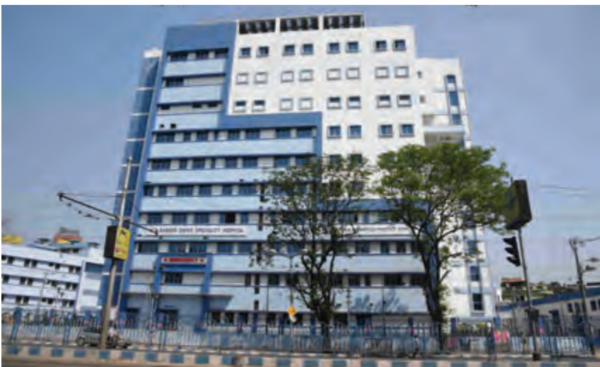
Shapoorji Pallonji E&C designed & built 18 Super-Multi-Specialty Hospitals in various districts for the Govt. of West Bengal. The combined capacity of these hospitals is 5,500 beds
