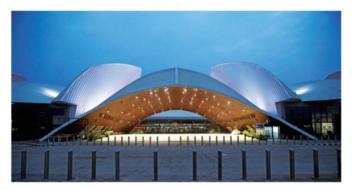
About 325 roof trusses were fabricated offsite at a fabrication facility at Delhi. This ensured that the roof trusses were fabricated and ready by the time the substructure works were completed. About 770 fabricated segments were then transported to the site before being assembled and erected at heights ranging from 10m up to 30m.
