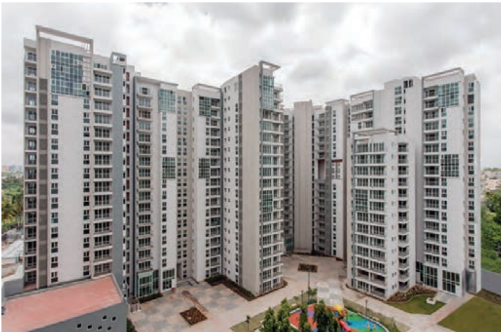
Monolithic concrete construction using aluminium formwork allows faster cycle times and reduces the requirement of construction labour and material wastage. Mass housing projects can be completed faster with better quality and safety as compared to conventional construction methods.
